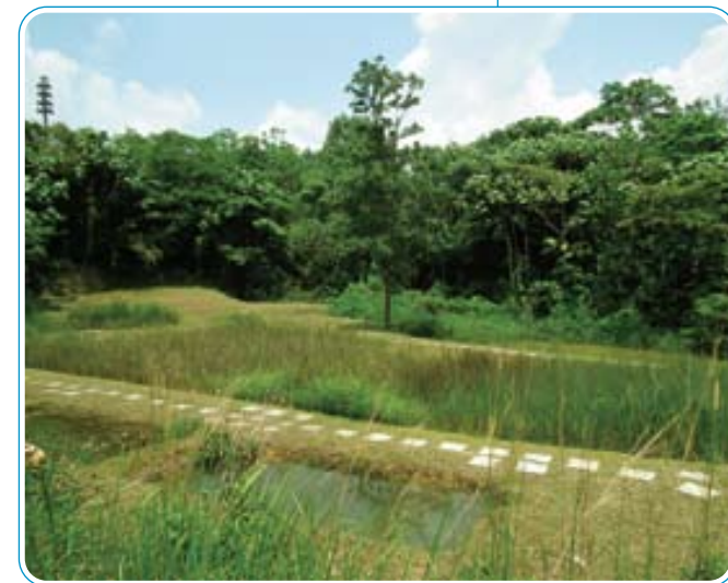
Project site after conversion to constructed wetland with well established wetland plants.
