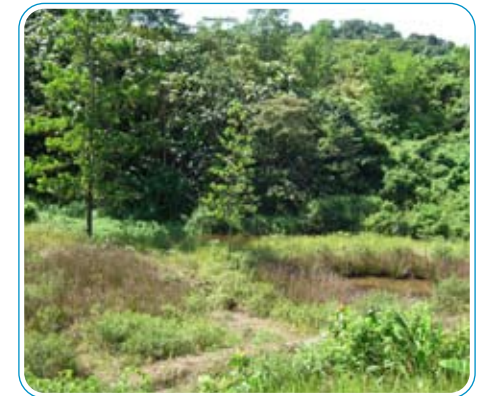
Condition of project site before conversion to constructed wetland. There were 3 small wetland cells which were silted up and overgrown with grass and invasive wetland plants.
